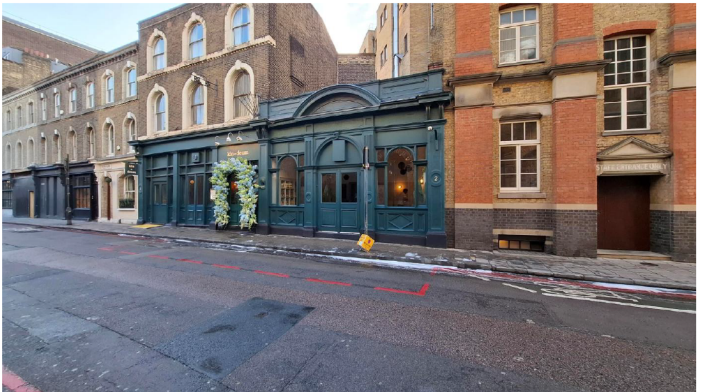
Pavement and road drenched with bleach water everyday
